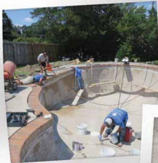
crack repair
