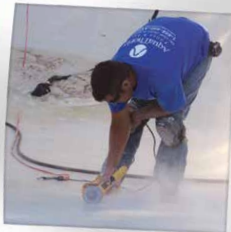
grind-out crack
