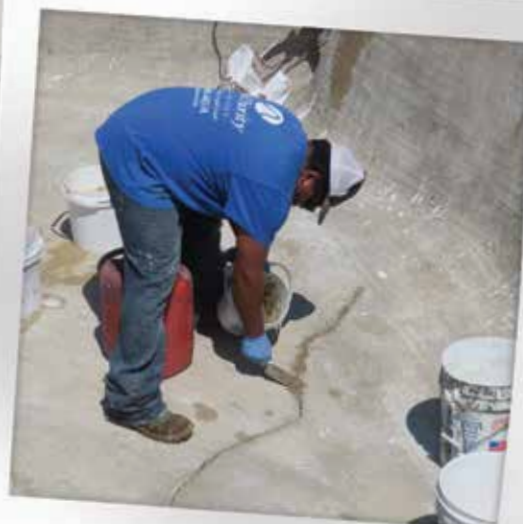
crack repair
